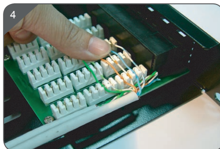
■ Arrange the wires according to the color code.
