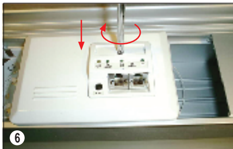
6. Assemble the central frame
